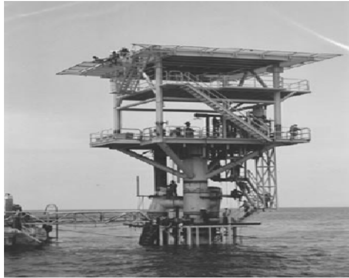
Figure 2.2 KARTINI – Braced Caisson Concept
