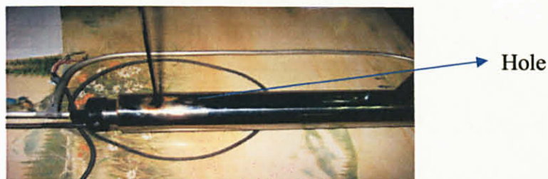
Figure 20: A Hole Drilled At The Bottom of The Jacket
