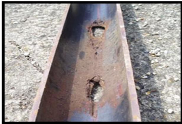
Figure 2: Damage in pipeline surface
