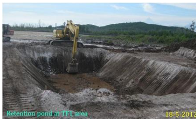
Figure 6: Retention Pond Development
