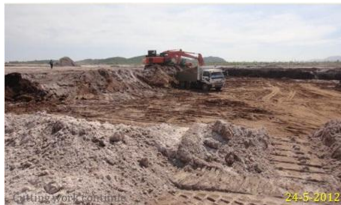
Figure 8: Cutting Work Activities
