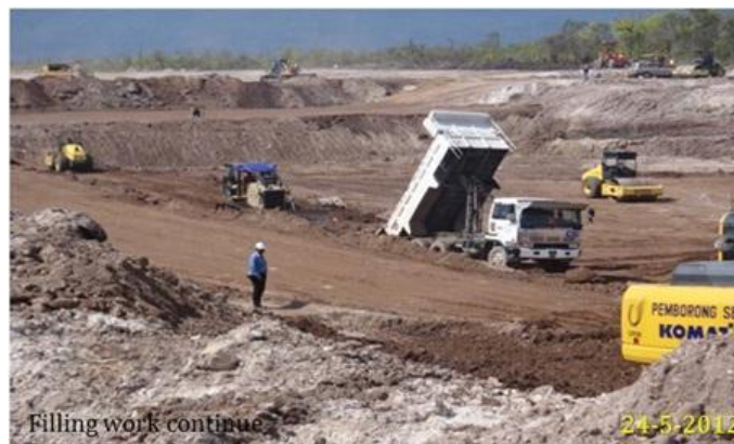
Figure 9: Filling Work Activities
