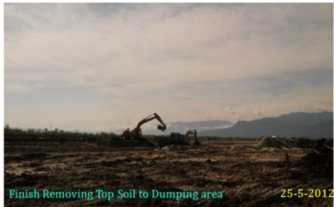
Figure 4: Top Soil Removal
