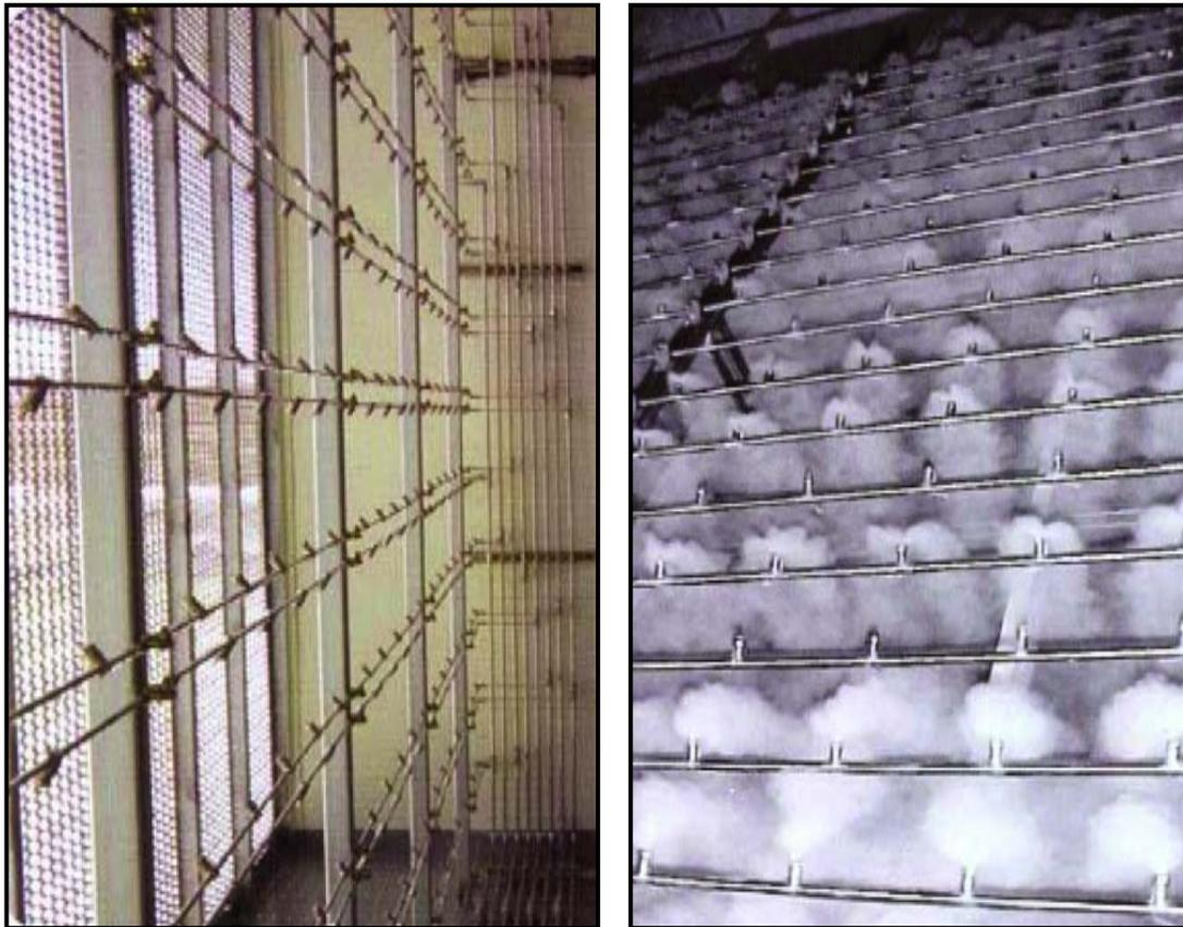
**Figure 2.12:** Mist of water form fogger nozzles [8]
