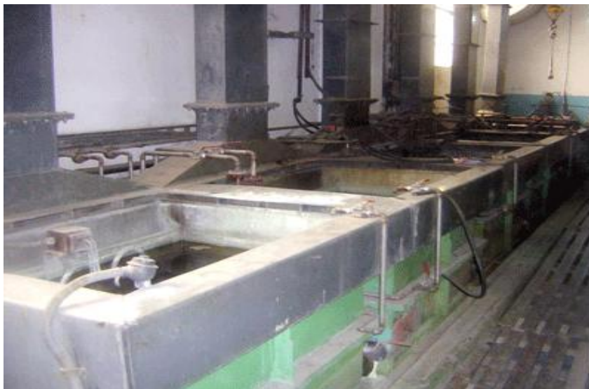
Figure 3: Hard chrome plating plant
