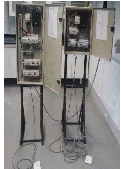
Figure 20: Two Distribution Boards
