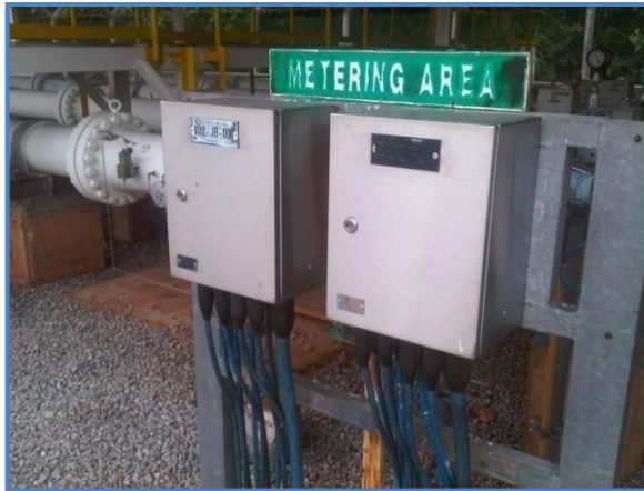
Figure 1-1: Metering area in Metering Station
