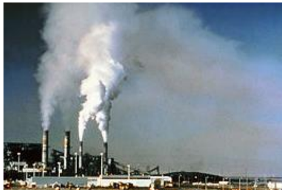
Figure 2.2: Flue Gas Emission through Stack Chimney
