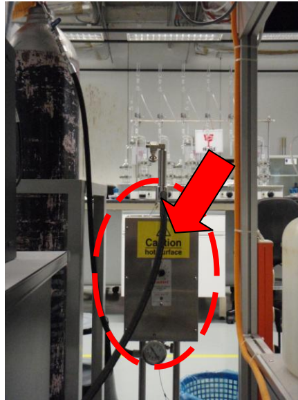
Figure 3.6: Dehumidifier: HPHT with Silica Gel inside
