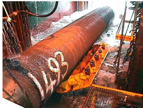
**Fig 2.1: S-Lay linepipe illustration (Left) and the linepipe move into the stinger**
