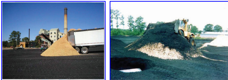
Figure 2.3 & 2.4: Unloading of Biomass and Mixed with Coal
