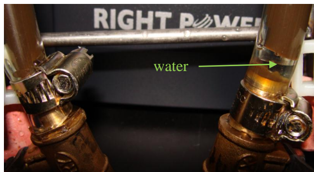
Figure 12: Water present inside the tube.
