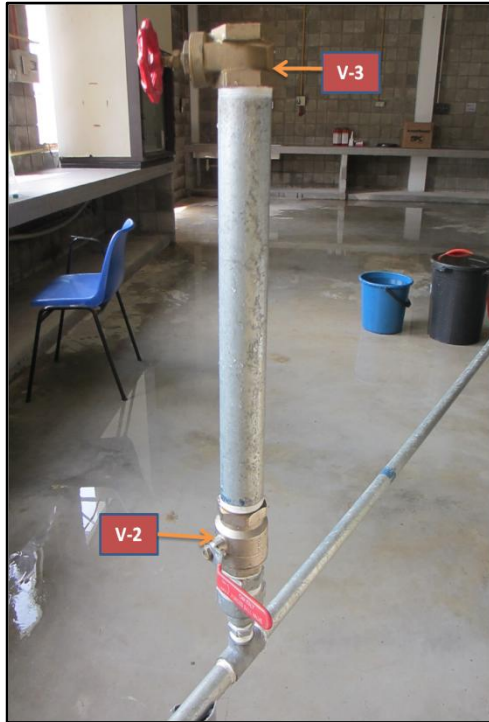
Figure 9: DRA Injection point
