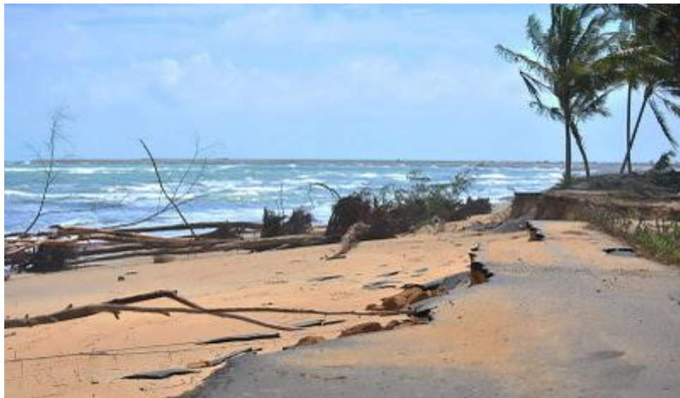
Figure 9 : Severe erosion at Teluk Lipat in December, 2011 ( Source : http://malaysiakini.com.my/ )
