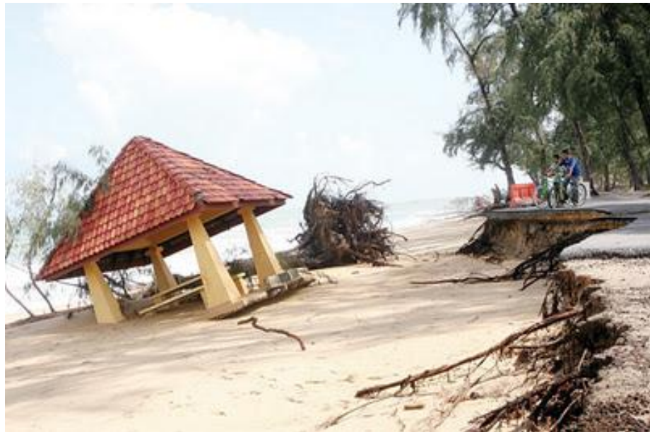
Figure 8 : A collapsed hut as a result of erosion at Pantai Rhu, Kuala Terengganu. (Source : http://www.kosmo.com.my/ )
