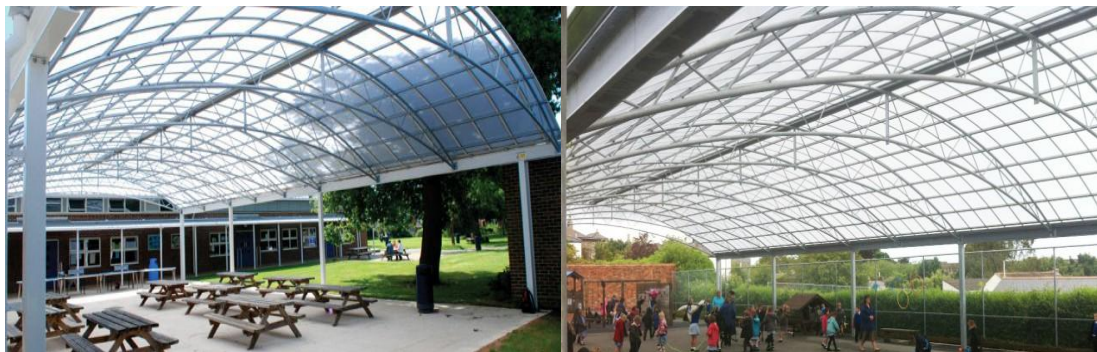
Figure 2.2 Steel canopy structure (sources: fordingbridge, 2012)
