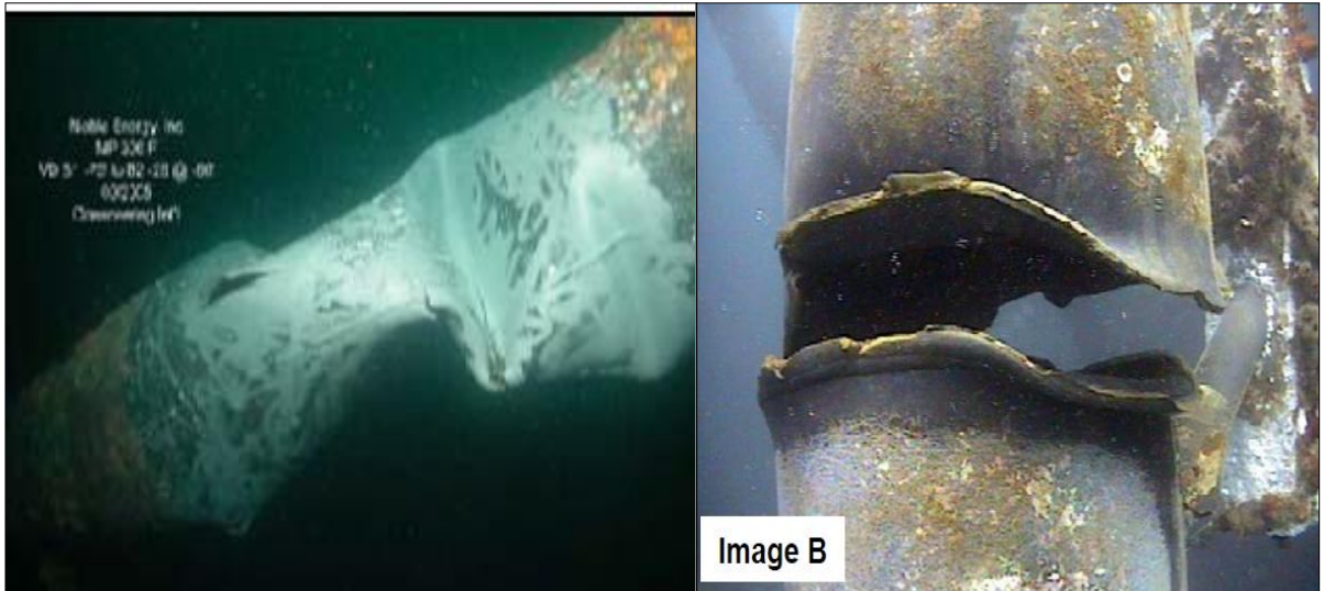
Figure 4 Brace damage (Energo Engineering, 2006)
