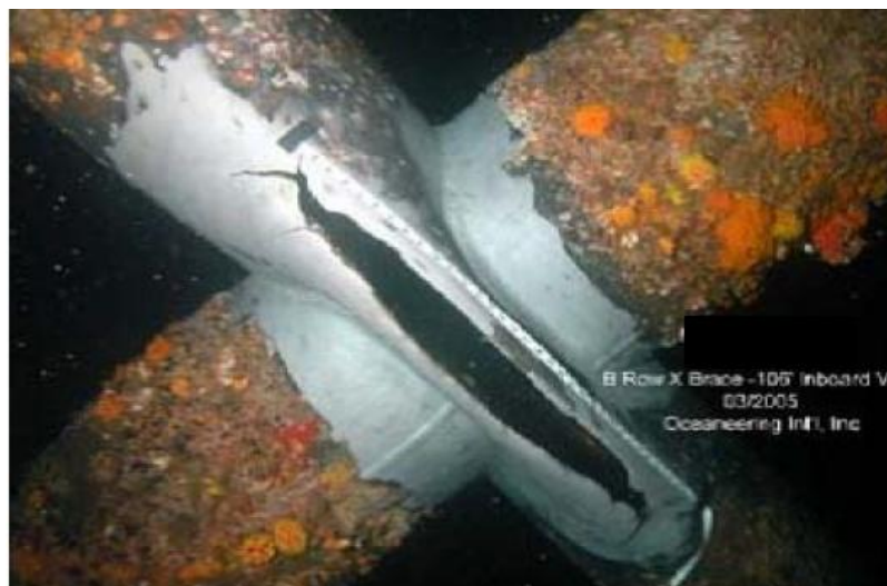
Figure 5 Crashing on X-brace (Energo Engineering, 2006)
