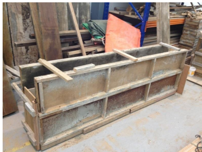
Figure 3-2: Contractors are doing formwork
