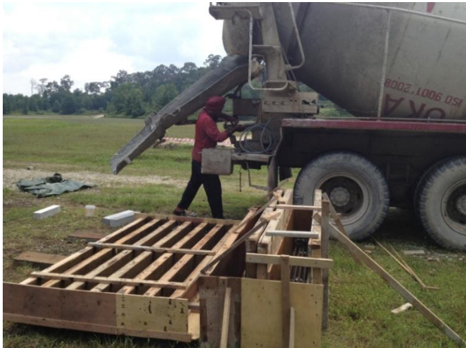
Figure 3-12: The concrete mix is ready to be poured into the formworks
