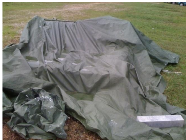
Figure 3-17: Beams have been covered with plastic cover
