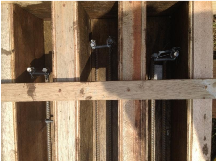
Figure 3-11: The position of reinforcement bars inside of the formwork
