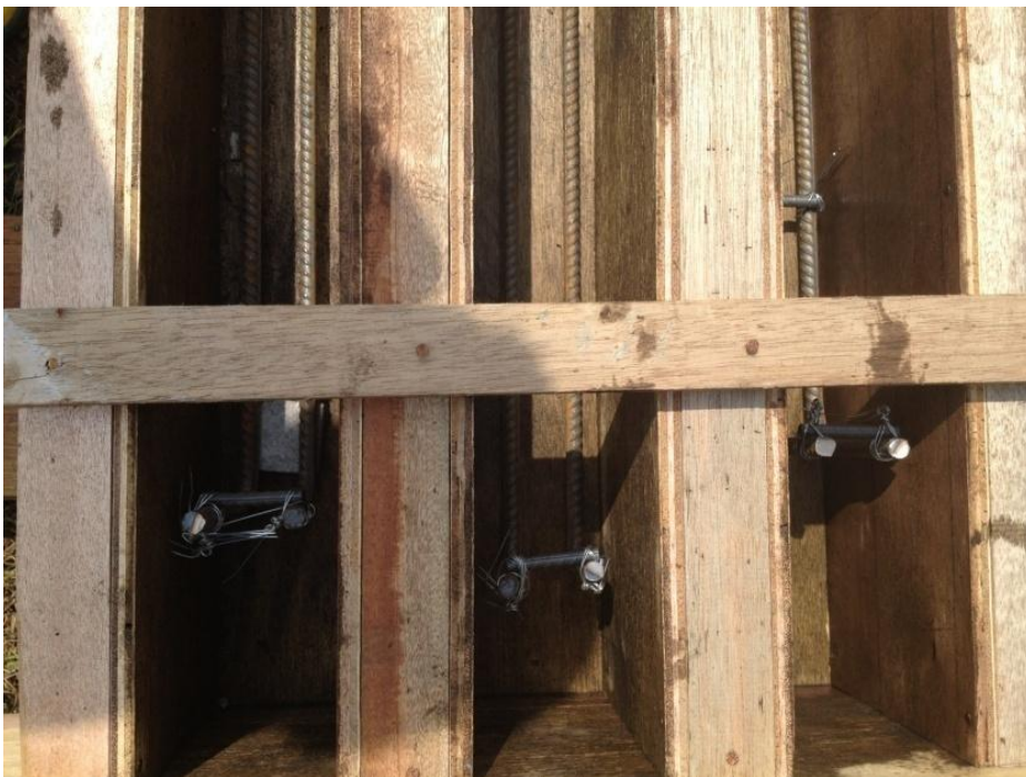
Figure 3-10: Grease applied to the formwork
