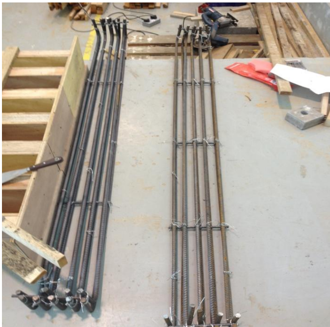
Figure 3-3: The reinforcement bars that have been bent
