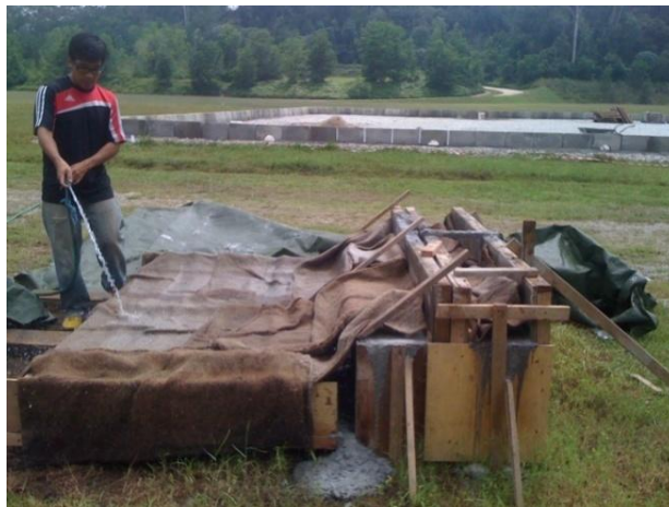
Figure 3-16: Gunny sacks are sprayed with water to make sure they becomes damp
