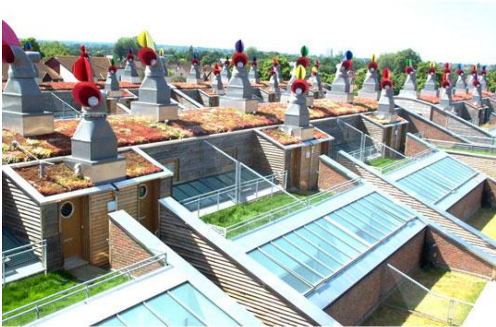
Figure 3 : The Advanced Green Technologies used in BedZED
