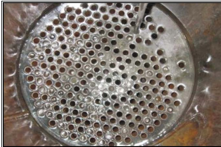
Figure 5: Salt deposits in the de-ethanizer reboiler top tube sheet after cleaning (Crew Energy Inc., 2011)
