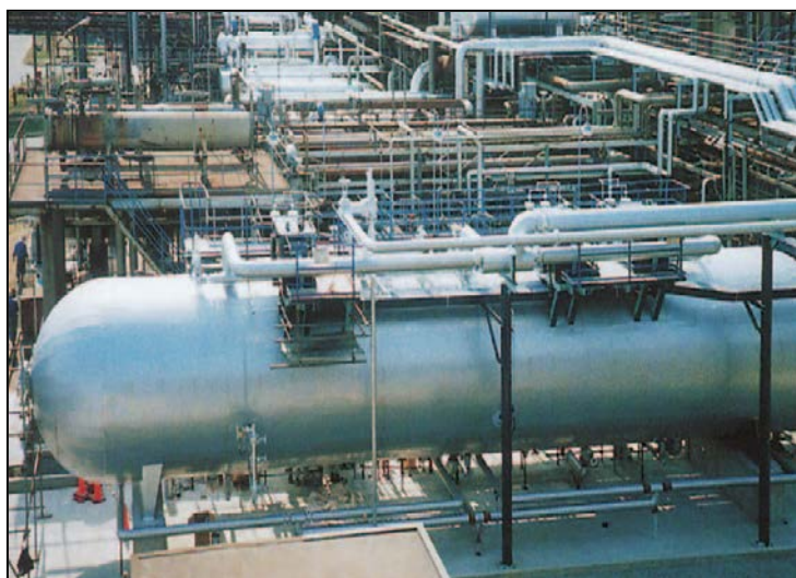
Figure 7 : Desalter (Cameron Inc., 2010)
