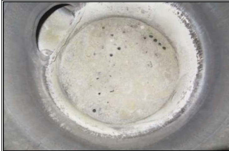
Figure 4: Salt deposits in the de-ethanizer reboiler top tube sheet before cleaning (Crew Energy Inc., 2011)
