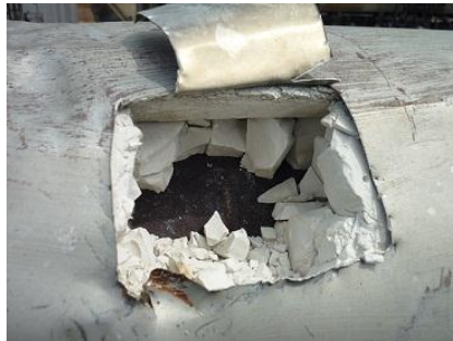
Figure 2.1: Corrosion Under Insulation [1]
