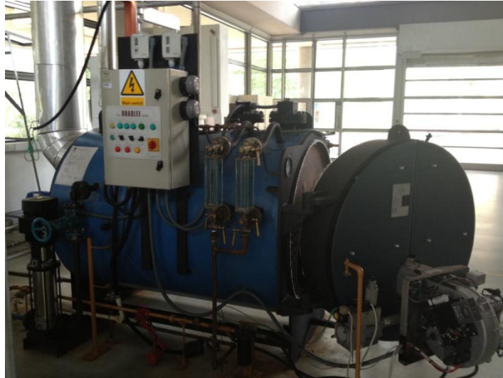
Figure 1.2: UTP Bradlee Steam Package Boiler
