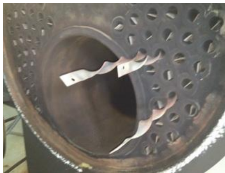
Figure 2.1 : UTP steam packaged boiler coil plate inserts
