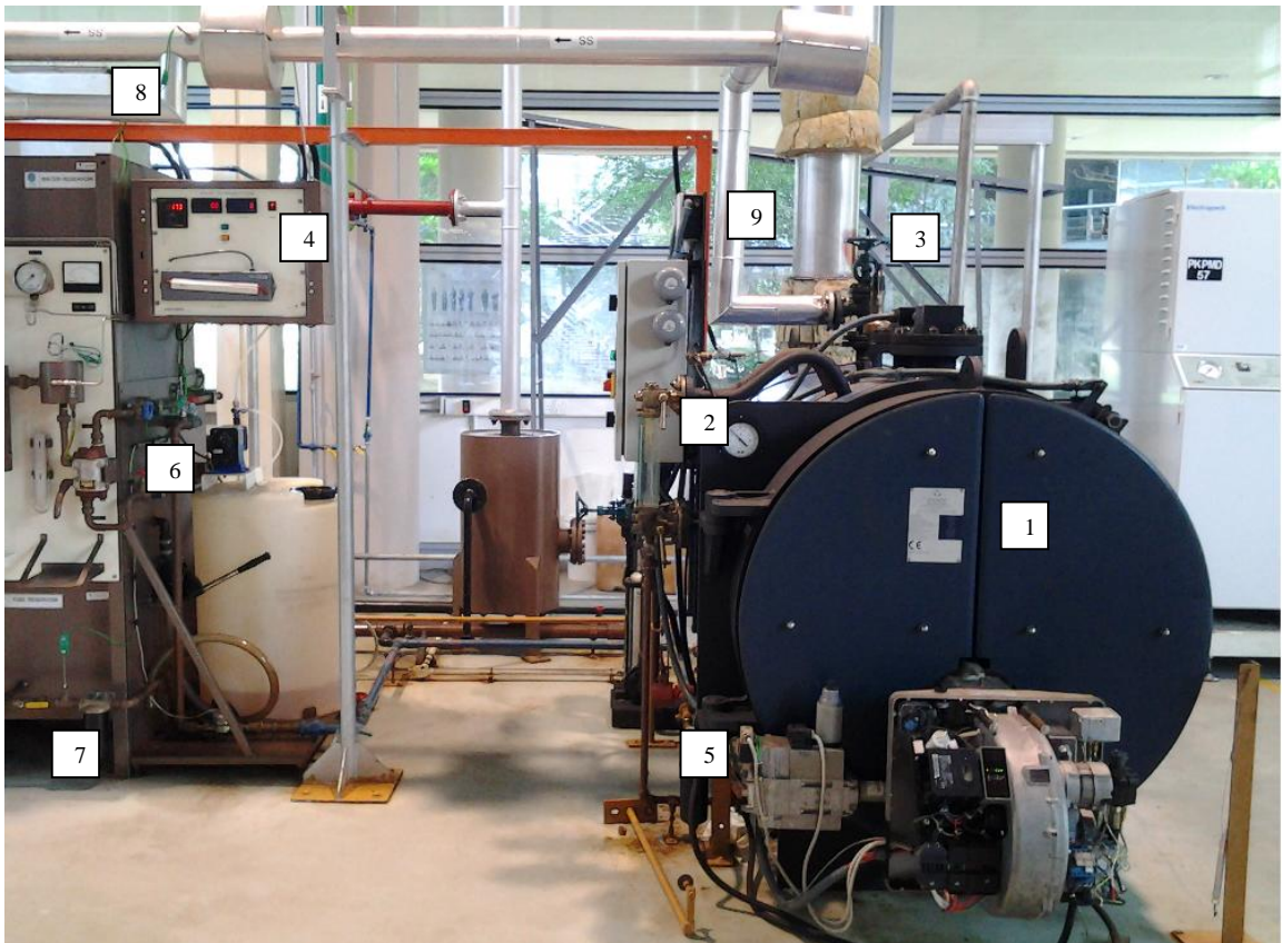
Figure 3.1: UTP Steam Packaged Boiler Instrumentation
