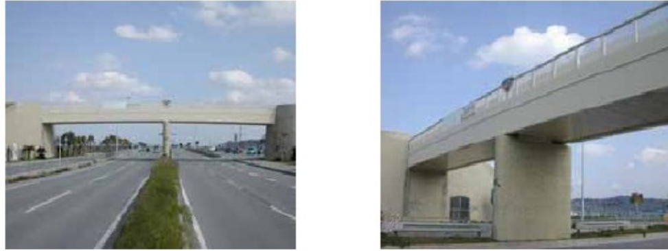
Figure 2.2: Pedestrian Bridge in Okinawa, Japan.
