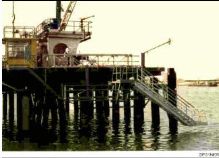
Figure A-5: Shore accommodation ladder (stationary system)
