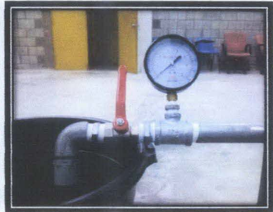
Pressure gauge configuration at the end of the test section
