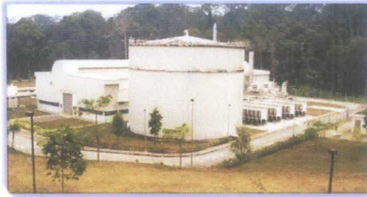
Figure 1 : Gas District Cooling Plant in UTP
