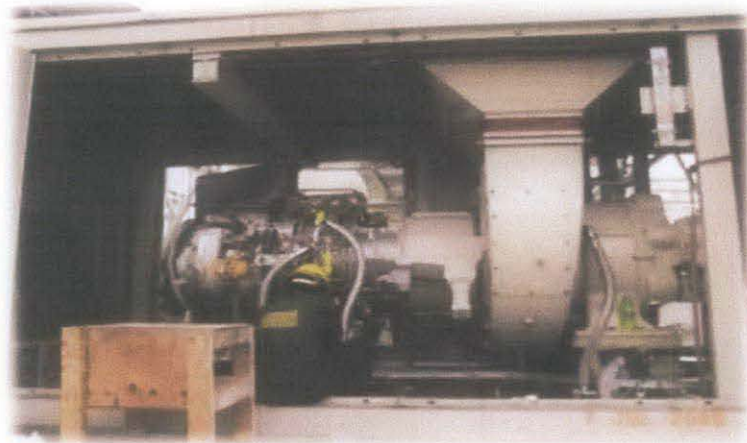
Figure 2: Gas Turbine during Maintenance
