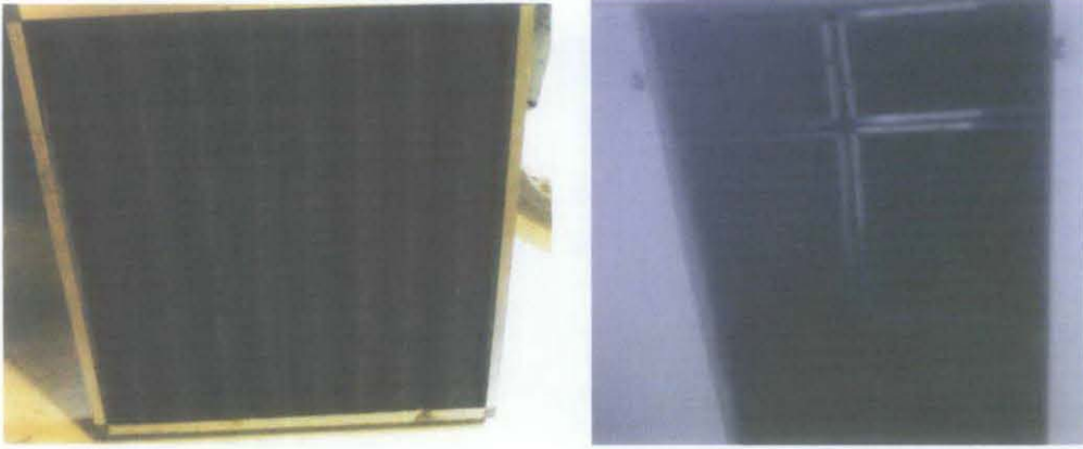
Figure 4.12 Current used filter image in AHU right wing building 18 level 3
