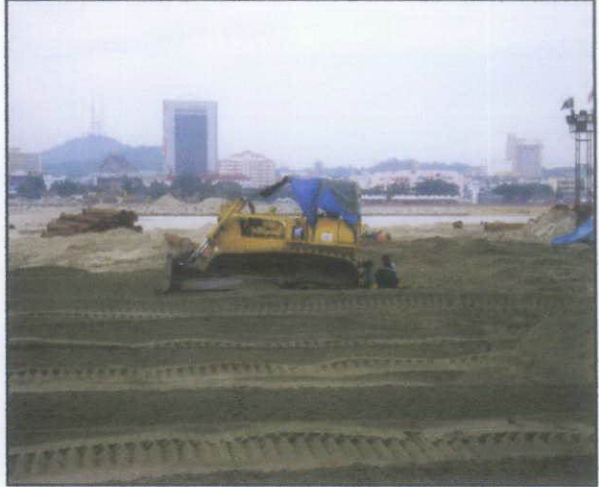
Figure 4.26 Completed reclamation area
