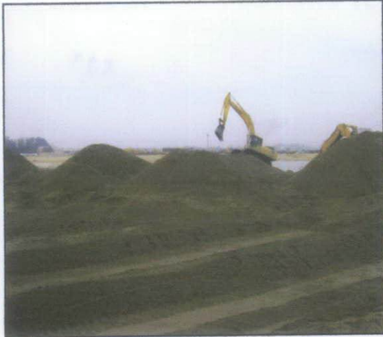
Figure 4.23 Excavator being used to level the sand
