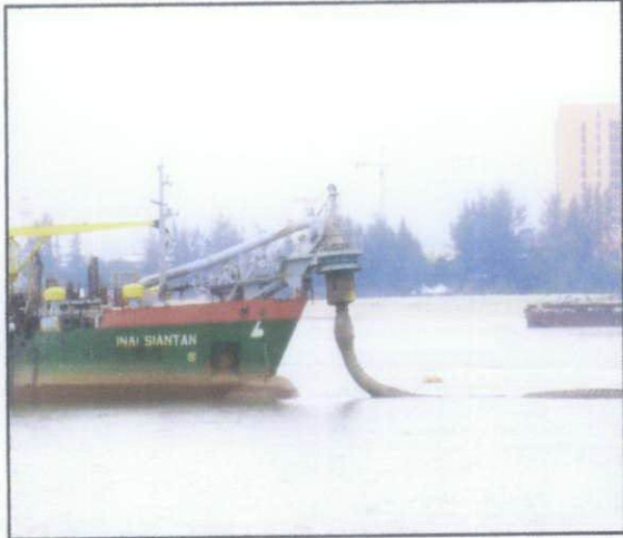
Figure 4.21 Sand being pumped out from the dredger
