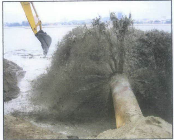
Figure 4.22 Sand being discharged at designated area
