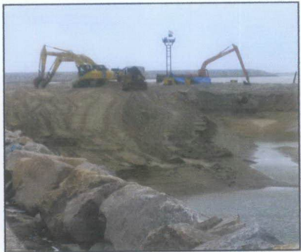
Figure 4.24 Ongoing levelling works
