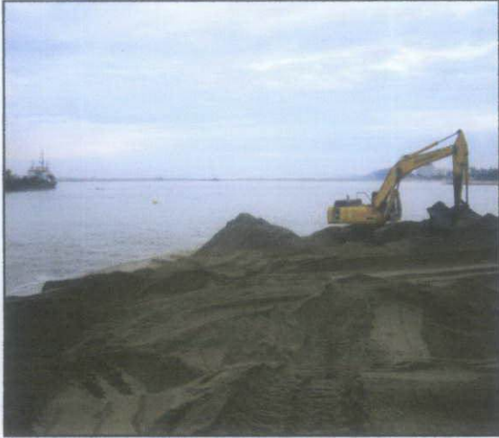
Figure 4.25 Excavator being used to level the sand
