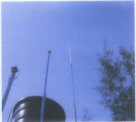
Figure 3.2 Base station, antenna and lightning conductor
