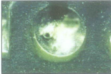
Figure 2: Blow Holes and voids
