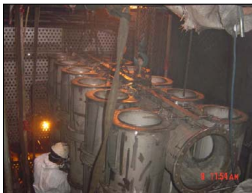
Figure 8: Installation Process of HID in V-1010 Production Separator
