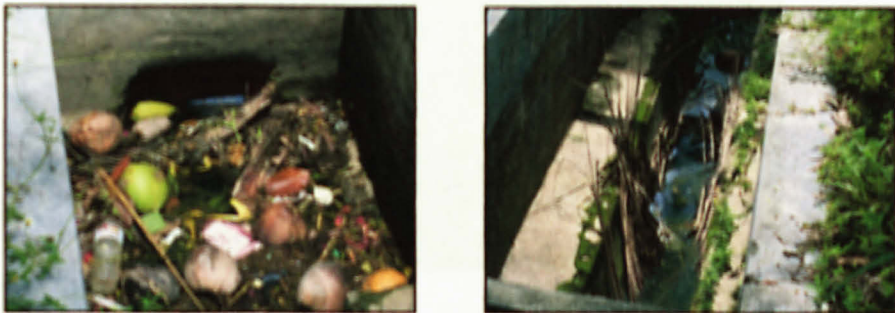
Figure 23: Clog/ Unmanaged drainage. Photos were taken from Taman Batu Gajah
