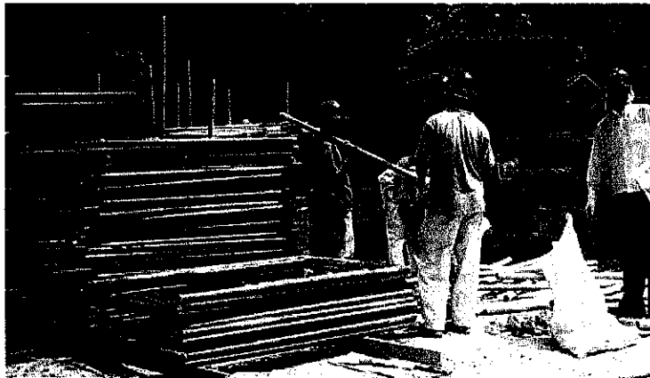
Figure 4.34: Efficient way of scaffold storage
