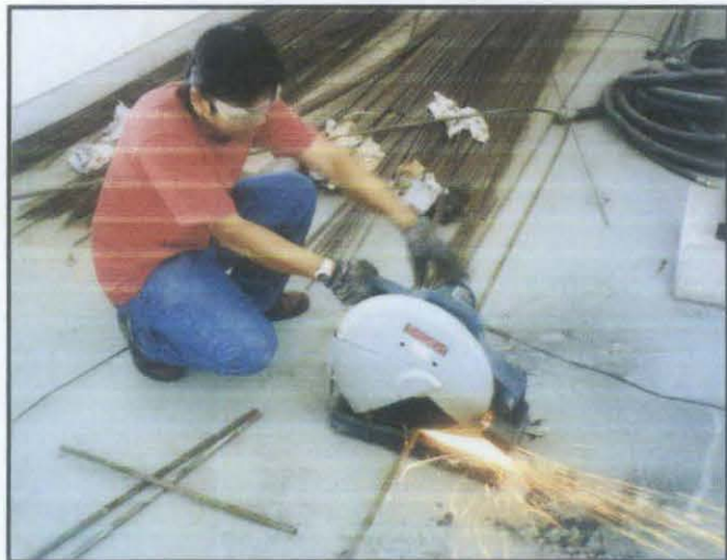
Figure 8 : Cutting steel bar into smaller pieces
