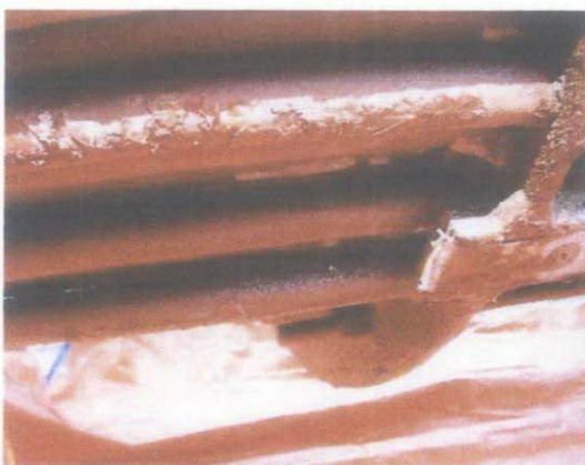
Figure 3.3: Coating damage and blister observed on E-105 tubing [6]
