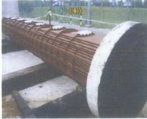
Figure 4.14: Touched-up peeled off coating after the contractor did hydro-jetting due to some damaged peeled off the existing coating [12]
