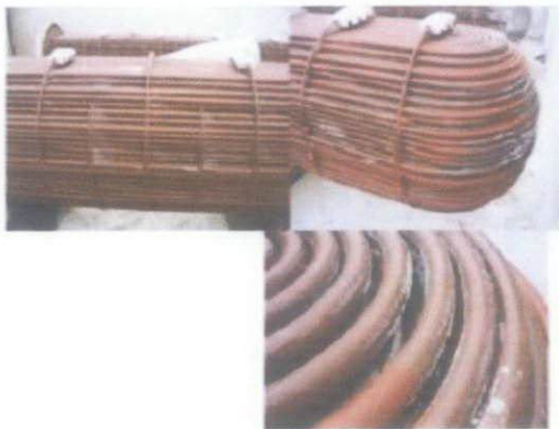
Figure 4.13: Peeled off coating in some areas due to water jetting [12]
