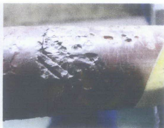
Figure 3.4: Close-up of E-105 localized corrosion/pitting and groove/mechanical damage near baffle plate to tube intersection [6]
