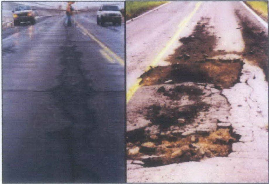
Figure 20: Fatigue from stripping problem and disintegration of pavement
