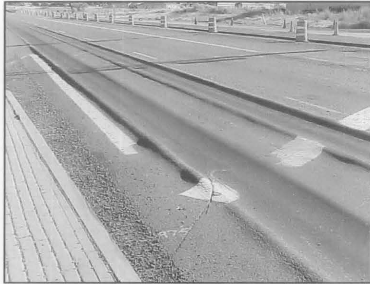
Figure 2.4 : Rutting from mix instability
