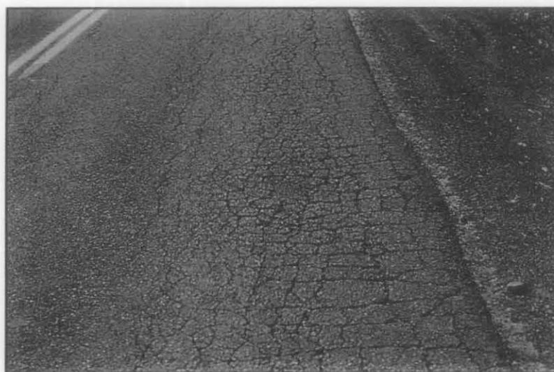
Figure 2.5 : Bad fatigue cracking
