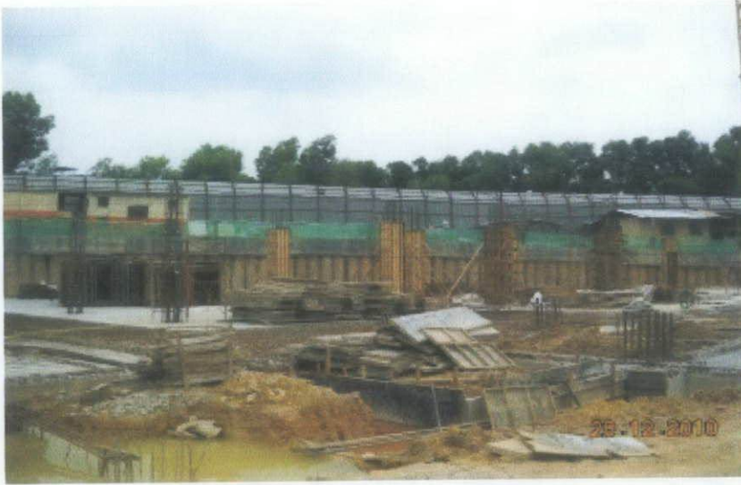
Basement 2 Columns being erected at Zone 4
