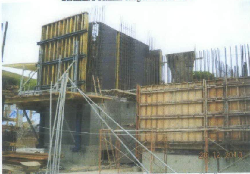
Basement 2 Lift Core Wall at Zone 1 is 40 % Complete (Hotel)
