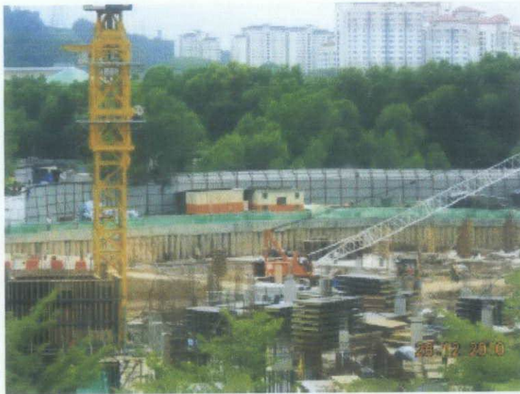
Overview of Project Site: View 1
