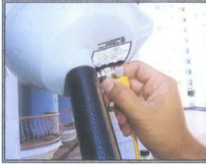
Figure 43: Cable 1.6m is connected to the antenna. Make sure that it is connected correctly.
