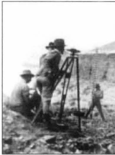
Figure 1: Conventional line-of-sight survey method: Early days levelling survey party ( http://www.photolib.noaa.gov/historic/c&gs/theb1773.htm )
