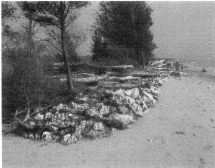
Figure 4.7 Gabion bund wall failures to protect pipelines
