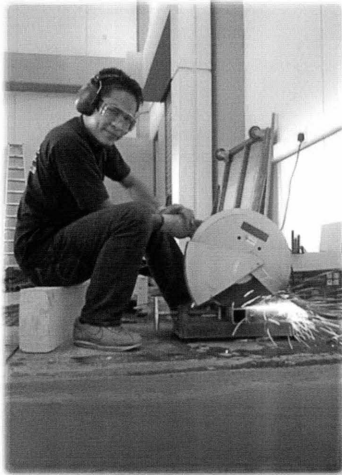
Figure A-3: Cutting Steel Tubes using Steel Cutter
