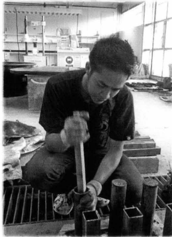
Figure A-5: Compaction of concrete using Compacting bar
