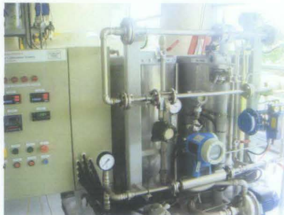
Figure 34: Overall Mobile Pilot Plant
