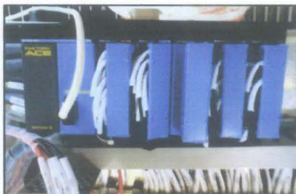
Figure 15: Programmable Logic Controller (PLC)
