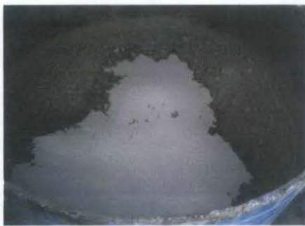
Mixing cement in the mixer
