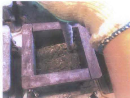
Placing concrete in moulds
