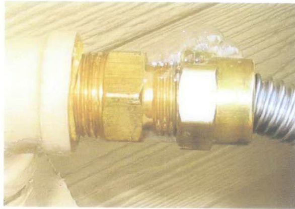
Figure 23: Example of Bubble Form in the Leak Test
