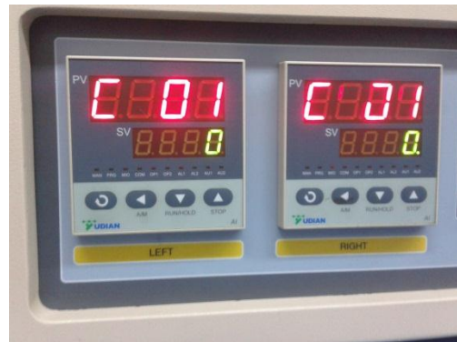
Key in the data at the temperature controller
