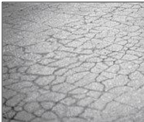
Figure 3: Fatigue Cracks
