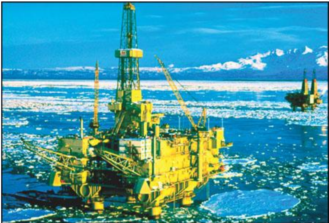
Figure 2: Steelhead Platform in Operation
