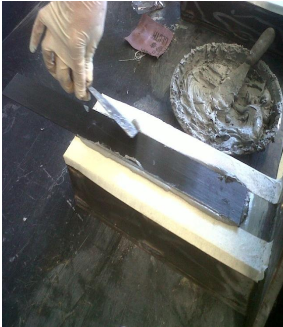
Figure 10. Applying adhesive on steel member
