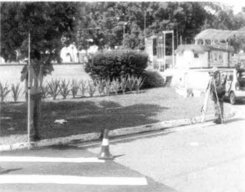
Figure 59: Measuring height using levelling technique
