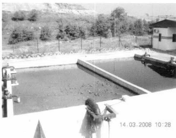
Figure 2: Flocculation and Coagulation Tank
